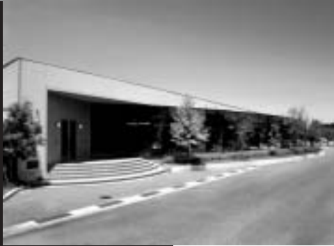
Photron USA's new HQ
